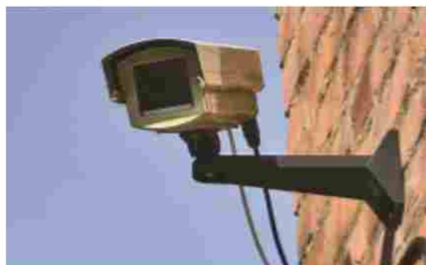
Figure 4.21: Closed-circuit television (CCTV) camera
