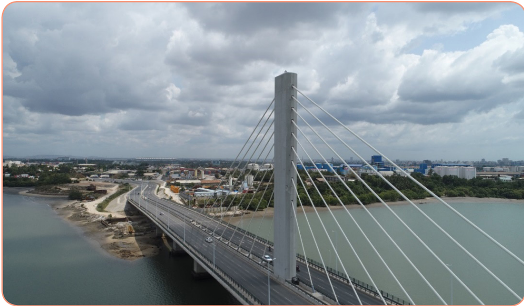
Figure 4.4: Nyerere Bridge in Dar es Salaam, Tanzania
