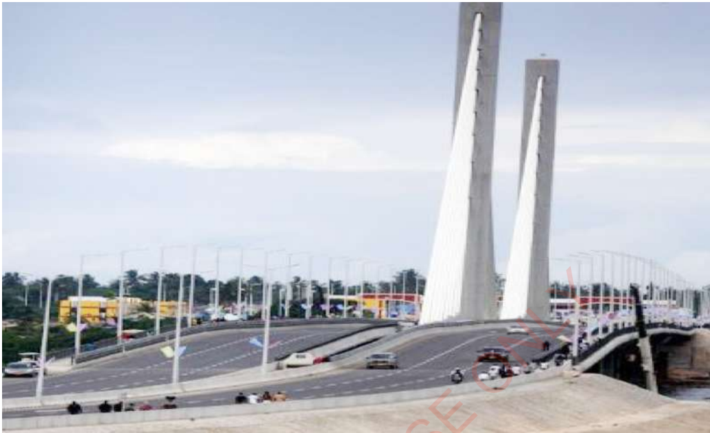
Figure 4.5: The Nyerere bridge in Kigamboni, Dar es salaam
